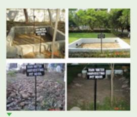
RWH system at API Chennai facility was also undertaken after a detailed feasibility study. The entire runoff rain water is connected to the rain water collection cum recharge tank of 2000 KL capacity and infiltration wells to recharge the ground water. The facility also has added a rain water recharging pit that collects rainwater from rooftops.
