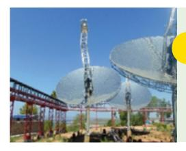
The paraboloid solar dish concentrator initiative that utilizes solar energy to preheat boiler feed water, at our facility is another step towards renewable energy use. The salient features of this initiative are maximum solar energy yield, high temperature delivery and reduction in the carbon footprint.
